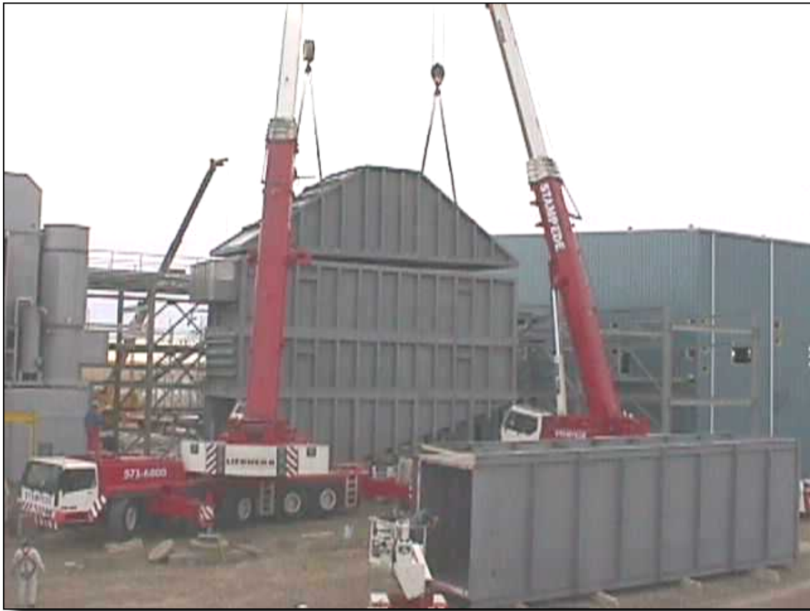
Figure 9: Simple Crane Work Required to Erect the OTSG Modules
