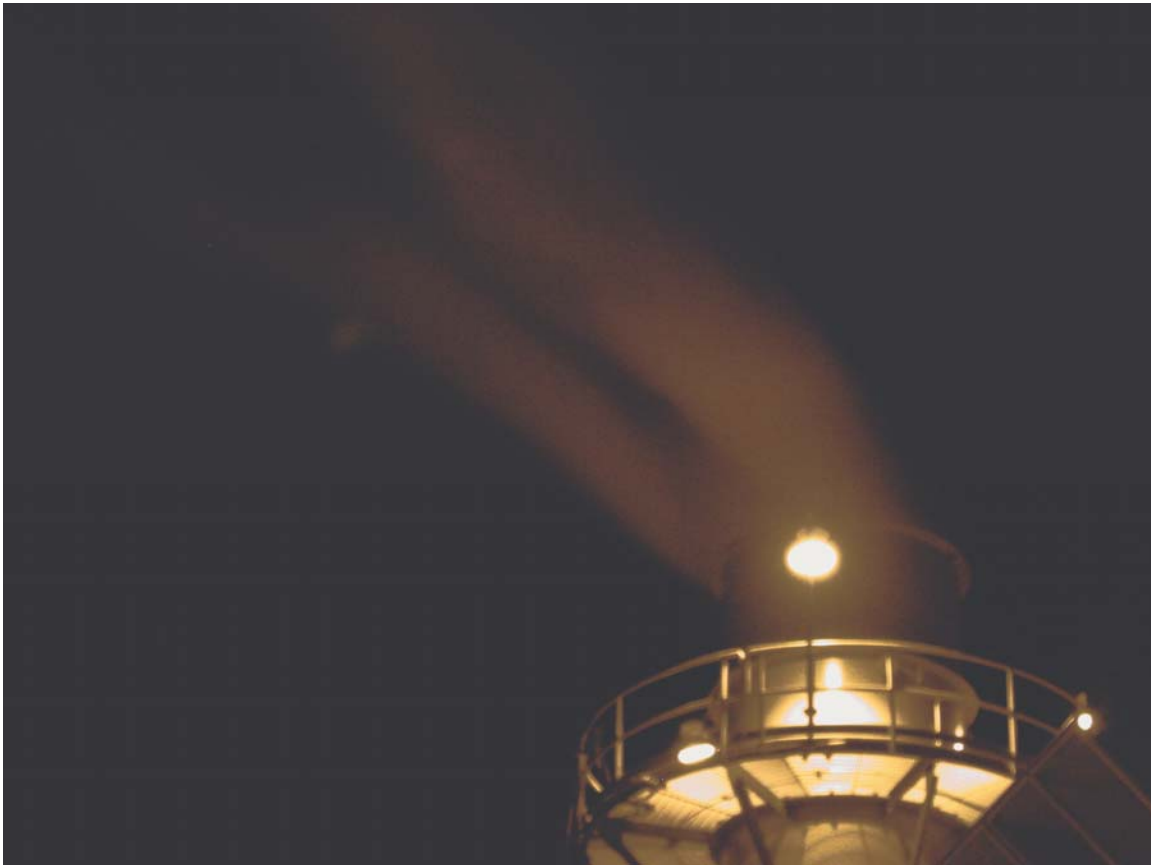
Figure #11 – Exhaust Stack of an OTSG During Soot Cleaning
