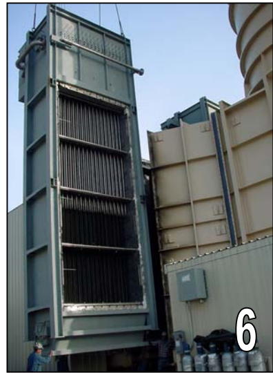
Figure #13 Steam Injection OTSG ® Erection Sequence
