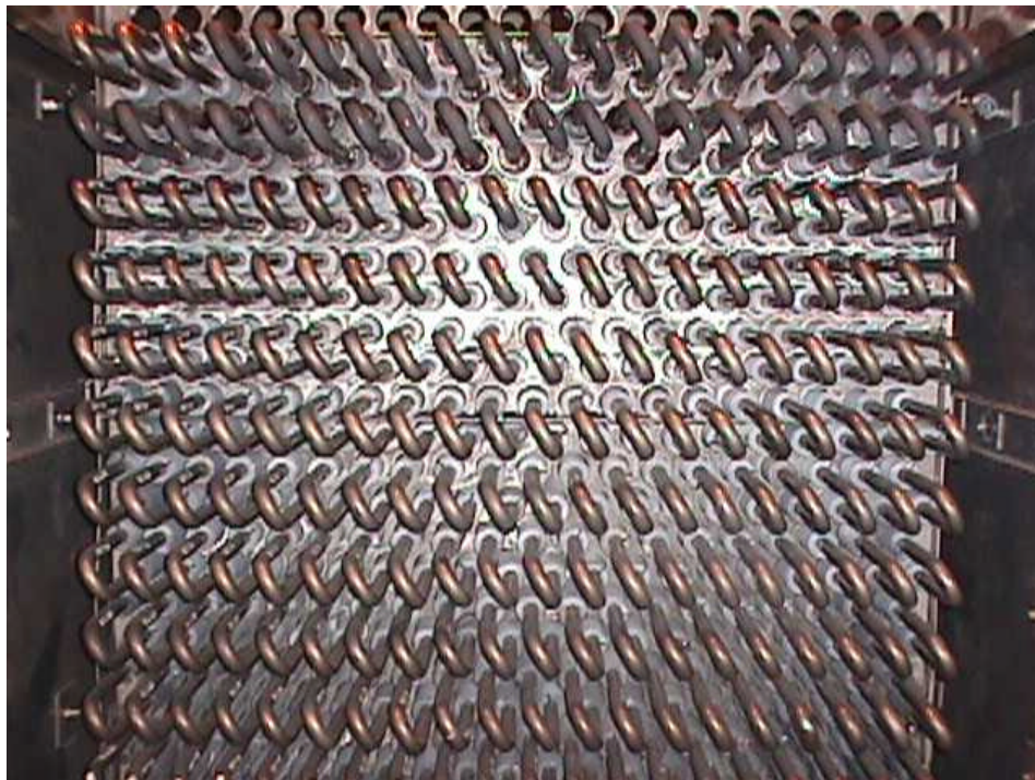
Figure 8; All u-bends and welds are accessible from the maintenance cavities on both ends of the OTSG. In the event of a tube, weld or u-bend failure, a circuit can either be brought out of service with a minimal impact on performance or repaired without causing damage to other tubes.
