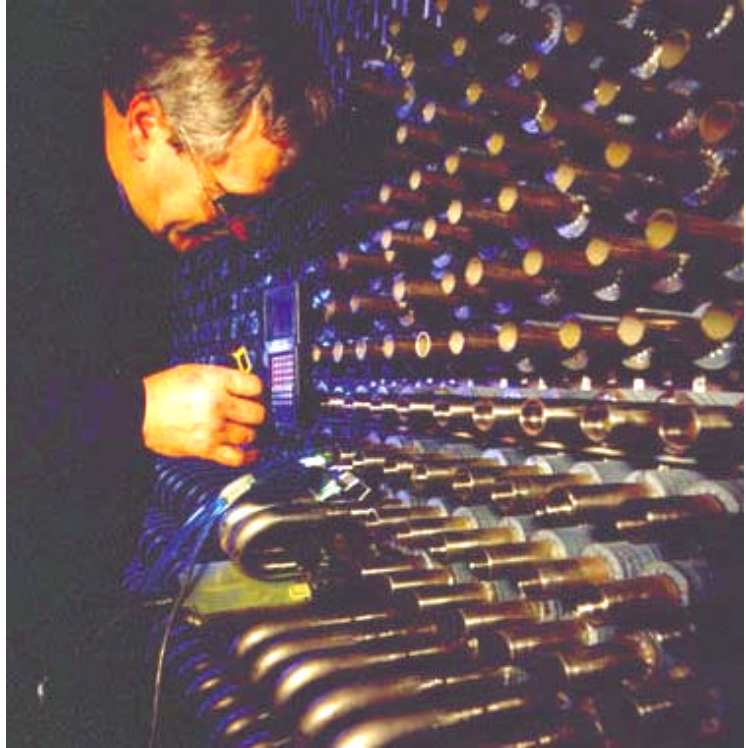
Figure 5; Orbital welding the u-bends to the boiler's tube bundle.
