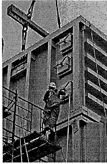
Figures 9, 10, & 11 OTSG installation sequence. OTSG's are easy to install. ASME Code welds inside the Section 1 pressure boundary are not required.
