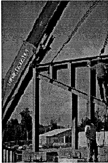
Figures 9, 10, & 11 OTSG installation sequence. OTSG's are easy to install. ASME Code welds inside the Section 1 pressure boundary are not required.
