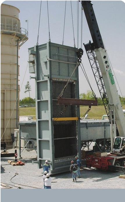
Once Through Steam Generators (OTSGs) were chosen by Calpine for installation in their first Gas Turbine steam Injection (GTI)/(STIG) simple cycle peaking plant located in Gaffney, South Carolina. The first phase of the project included the GTI retrofit and installation of OTSGs on units 1 through 3. The second phase of the project included the GTI retrofit and installation of OTSGs on units 4 and 5.
