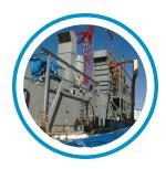
IST was contracted to supply one (1) OTSG for the Pinelawn Combined Cycle Plant. The OTSG was built with an HP steam circuit, supplemental burners fired to 1340 F and SCR and CO systems for emissions control. The plant features one (1) x 43 MW LM6000 gas turbine and one (1) steam turbine.
