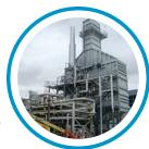
IST was contracted to supply two (2) OTSGs for the GTAA Combined Cycle plant. The OTSGs were built with HP and LP steam circuits, and also included supplemental burners, Provisional SCR and CO systems for emissions control. The plant also features two (2) x 43 MW LM6000 gas turbines and one (1) steam turbine.
