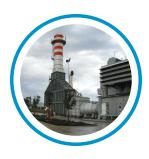
IST was contracted to supply one (1) OTSG for the ElettroGorizia Combined Cycle plant. The OTSG was built with HP and LP steam circuits. The plant also features one (1) x 43 MW LM6000 gas turbine and one (1) steam turbine.
